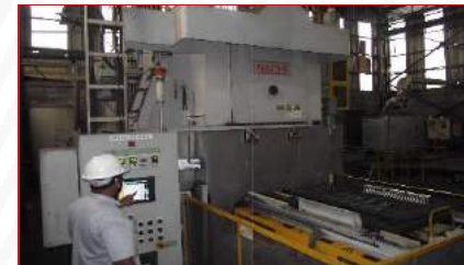
FASILITAS VACUUM CARBURIZING (1 UNIT)
